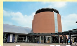
Main building of the Kitsuregawa Rest Area
